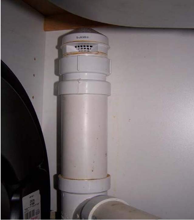
Photo 4: Air Admittance Valve
