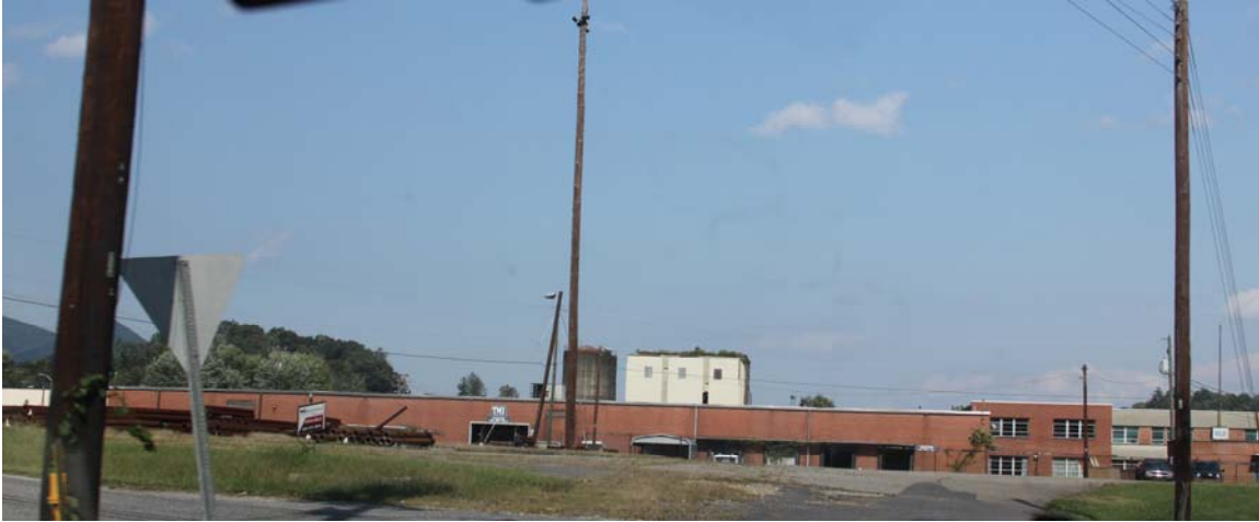
Old Fort Finishing site
