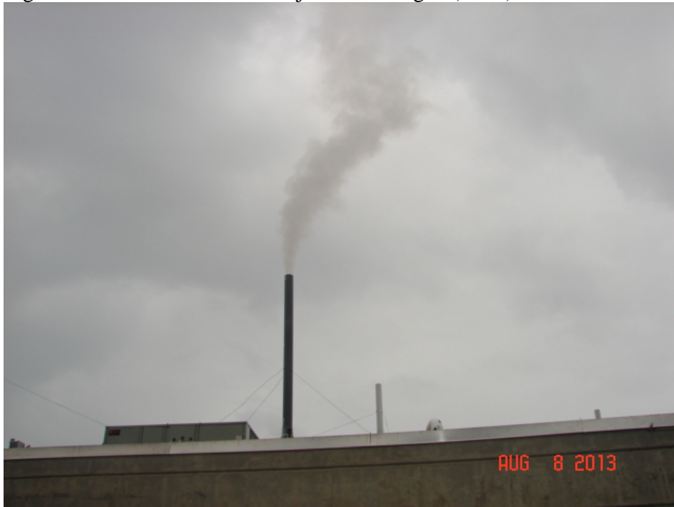
Figure 3: Exhaust from Total Kjeldahl Nitrogen (TKN) Exhaust Stack
