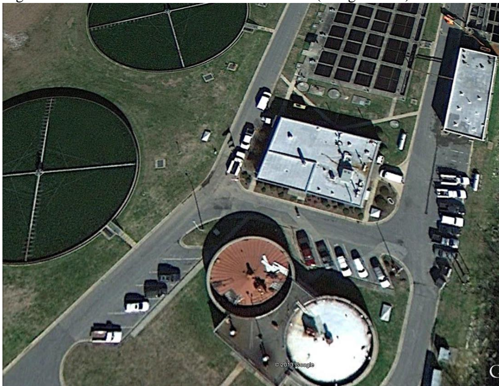
Figure 4: Asheboro Wastewater Treatment Plant (Google Earth)
